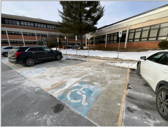
OVERVIEW OF ACCESSIBLE PARKING AREA
