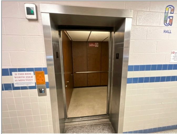
LOBBY LOOKING AT CABS
